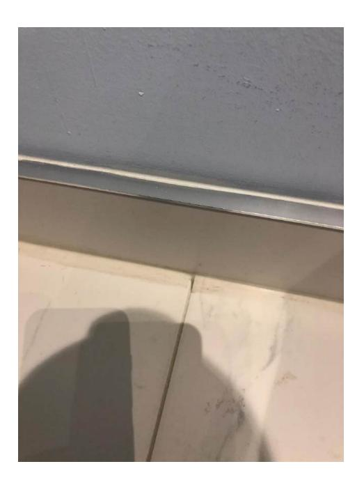
The floor tiles in the main floor powder room are mis-aligned with reference to the home's design; they should be perpendicular to the as-built configuration.
