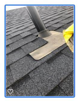
Formal cleanup is required at the metal junction flashings.
