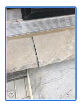
Patching and finish work is required at damage at the front left corner.
