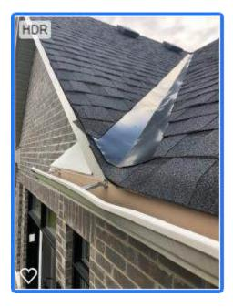
The roofing is incomplete at the end of one of the lower strip sections, at the bottom of a diagonal metal piece.
