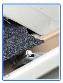
The metal junction flashing is incomplete and not sealed. There is a space between the angled part of the flashing and the horizontal part of the flashing. A formal, continuous and fully-sealed flashing must be provided by the builder. Also, two of the shingles are not fully seated at the left side low roof, as shown in the photo.
