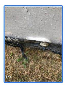
The membrane system has not been formally trimmed at basement windows. Such systems are normally trimmed formally below the window sills.
