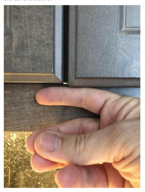
A gap is observable inside the kitchen drawers where the face piece meets the bottom section.
