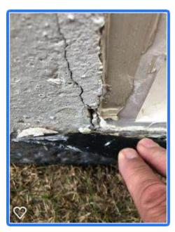
Debris is observable – and creates a gap – between the waterproofing membrane and the outside face of the foundation walls. The debris should be removed, as possible, and the top edge of the membrane should be formally fastened. (Note: for reasons unknown, sealing the top edge of membrane systems outside foundation walls is not required as per specifications.)
