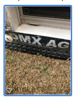
Informal parging material prevents formal caulking at the joints where the basement windows meet the foundation walls. All basement window joints must be fully and formally caulked.
