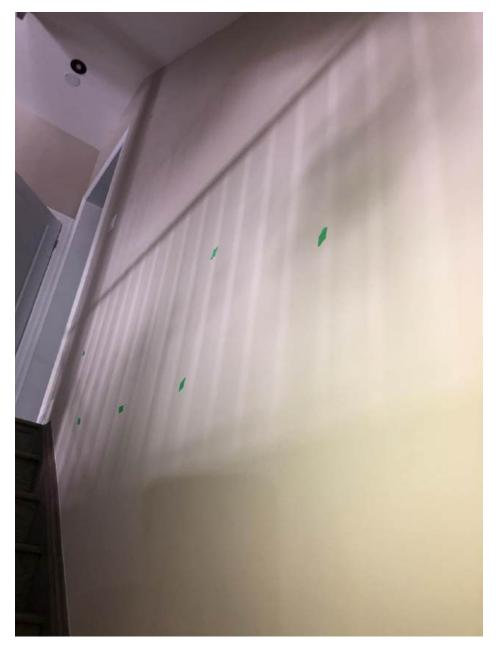
Final caulking is incomplete at the open joints at the junctions where the windows meet interior finishes.
