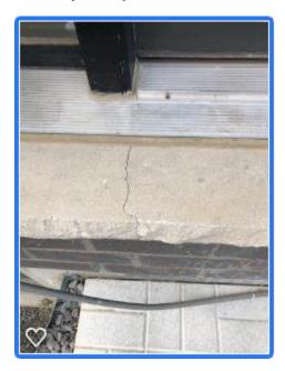
The mortar joint within the rear door sill should have been formally caulked.
