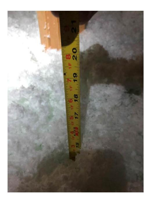
Further, there appear to be low spots above the middle part of the front second floor bedroom. Those low spots are observable from the access to the high attic. And, the thought that the spots might be low were confirmed by thermal camera readings in the middle of the bedroom. The lowest ceiling reading of 19.5 degrees C was found at the middle of the right part of the front bedroom. The builder should be invited back to the home to address this deficiency.
